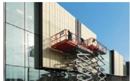
**Economic feasibility.** Perfect substructures guarantee efficient panel installation. The low panel weight offers advantages in terms of statics, transport and handling.
